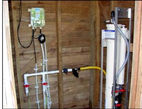
Contaminated water from the mountain stream is gravity fed under low pressure through the SkyHydrant water filter to produce safe potable water. The water is then pumped to two tap stands for easy access for the school children
