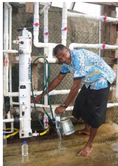
**Two SkyHydrant water filtration units can produce up to 20,000 litres of safe water per day**
