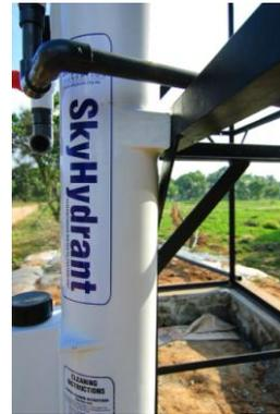
Tanks are mounted on high grounds to increase gravitation strength so that filtered water can be piped over a longer distance to the distribution point.
