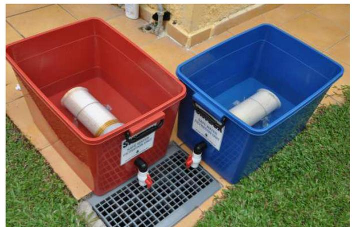
**Photo 1.0 / 2.0: locally sourced storage containers were adapted for the SkyBox™ membrane**
