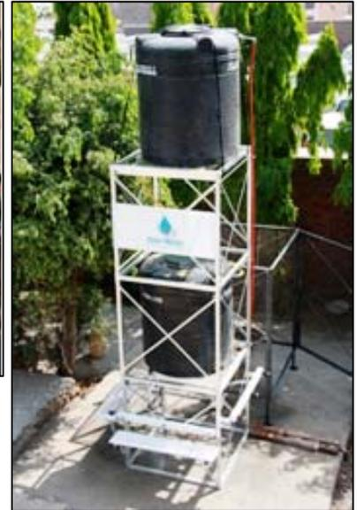
A SkyHydrant water purification unit and a SkyTower (including a hand wash facility) were deployed on site, providing safe water for all children and staff. The SkyJuice technology is appropriate and effective and most importantly, it is sustainable. There are virtually no ongoing maintenance costs; therefore the community is not burdened with expensive running costs.
